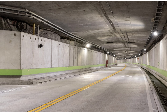
Oriente Tunnel Medellín - Colombia
